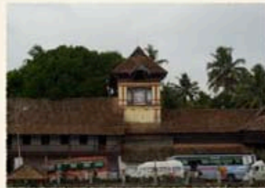
East Fort views; Clock Tower
